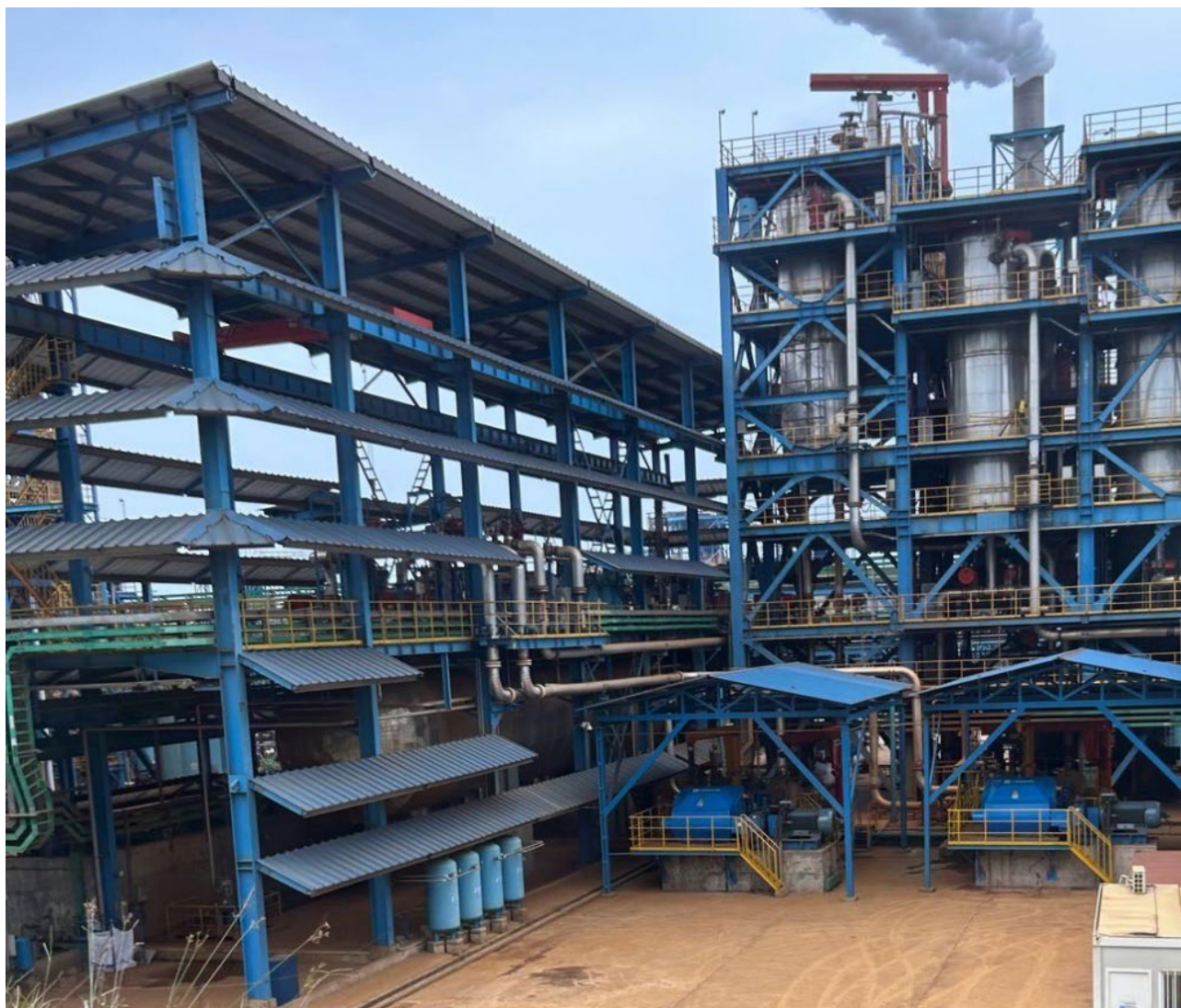
View of HNC operations
