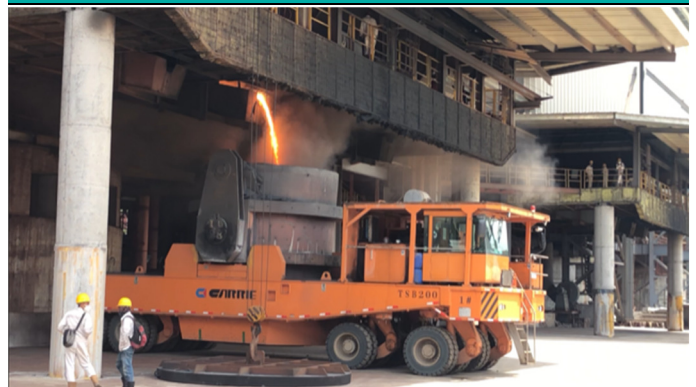
Figure 4 - NIC RKEF site March 2019 – Hengjaya lines
