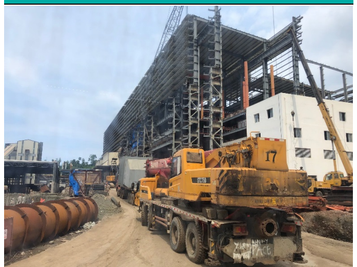
Figure 2 - NIC RKEF site March 2019 – Ranger lines in foreground
