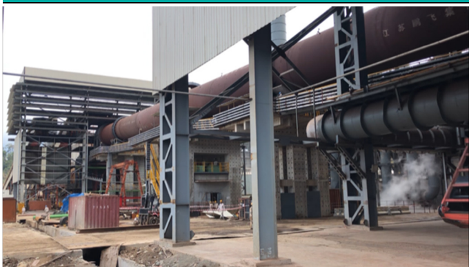
Figure 3 - NIC RKEF site March 2019 – Hengjaya lines
