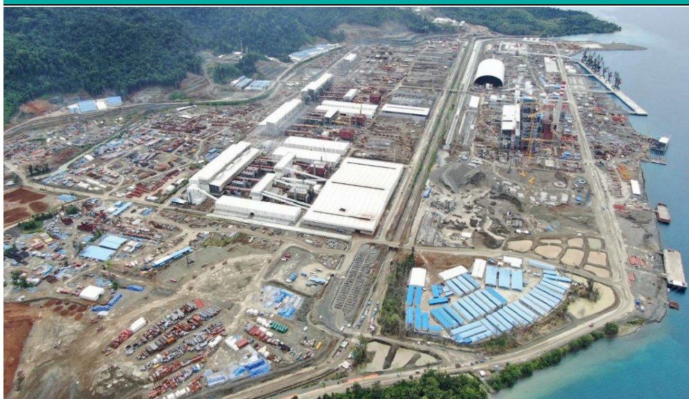
Figure 1 - RKEF lines at the IWIP - under construction
