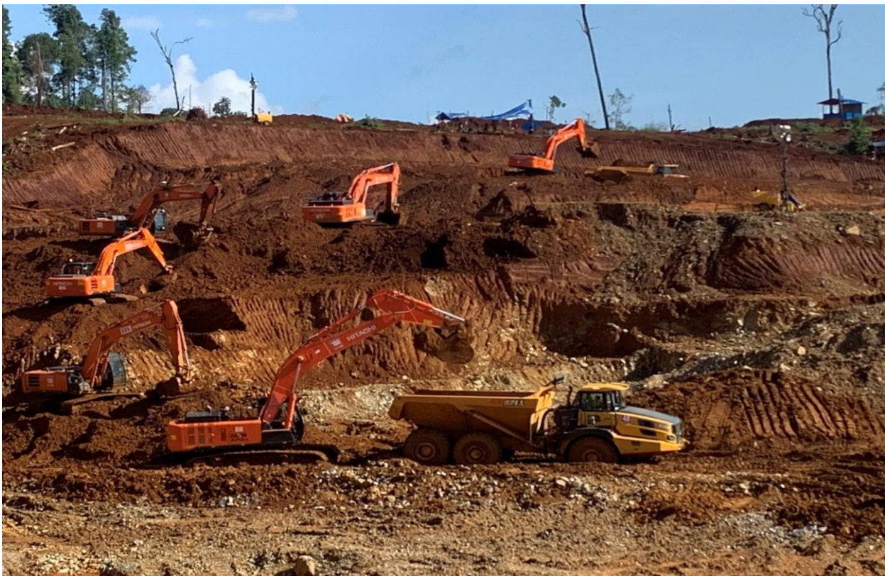
Central Pit – July 2020.
