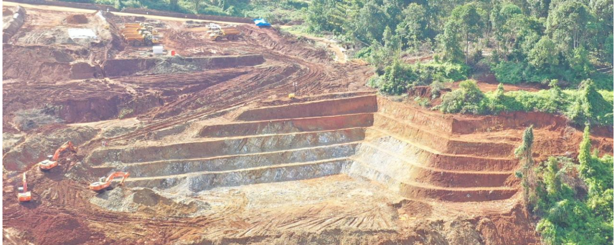
Civil works for ore scalping (Ore tiphead).
