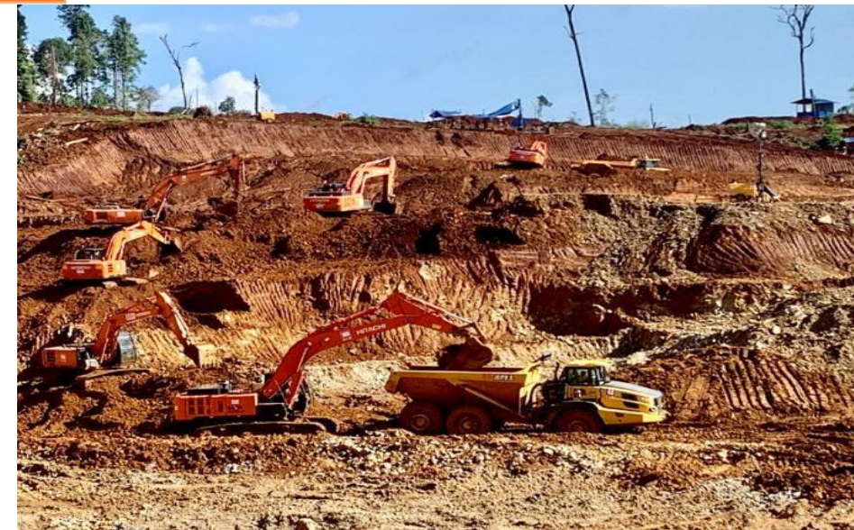
Central Pit – July 2020
