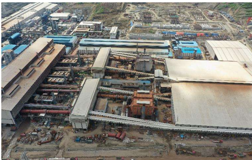
Aerial image of Nickel Mines 60% owned Hengjaya Nickel and Ranger Nickel
