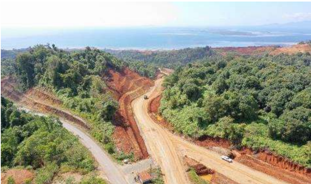
Widening of existing haul roads for larger haul trucks almost complete.
