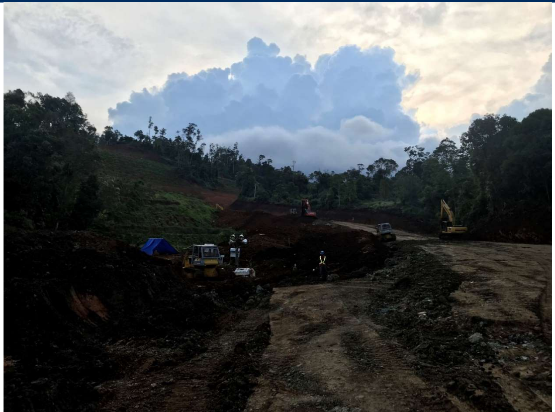
Figure 6: Road Under Construction from Hengjaya Port to Central Pit (March 2019)
