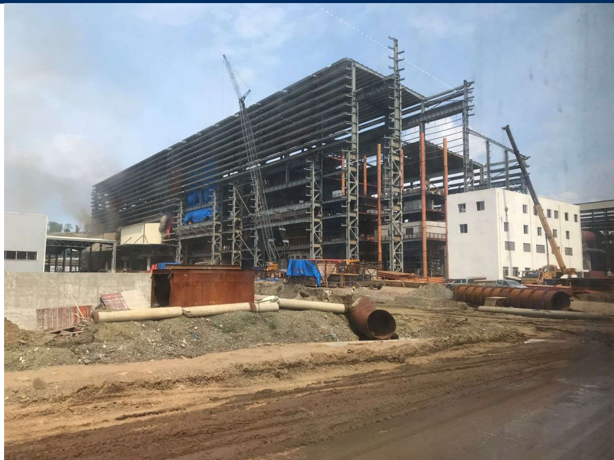
Figure 14: Ranger Nickel RKEF Lines Under Construction (March 2019)
