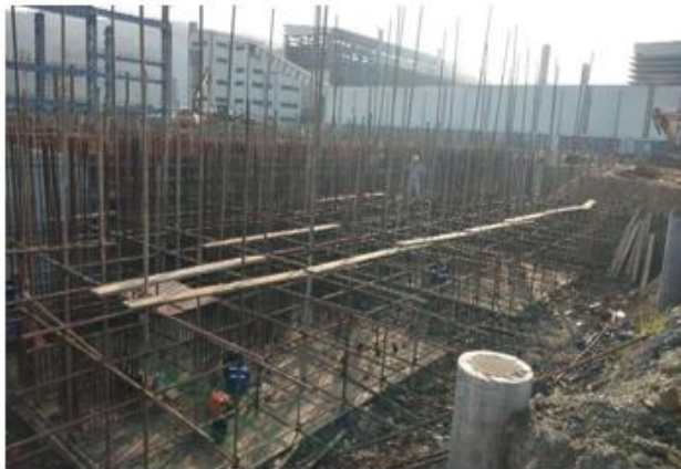
Scaffolding support for the RKEF Lines
