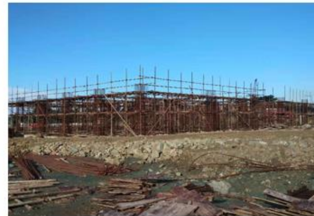
Column reinforcement for Electrostatic Precipitator
