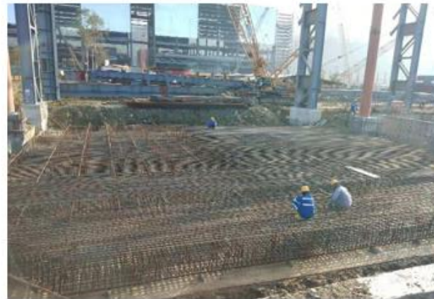
Foundations of Main Workshop
