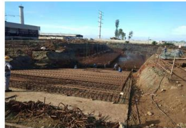
Foundations for Dry Ore shed
