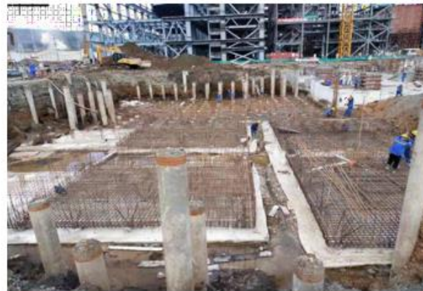
Foundations for ANI powerplant
