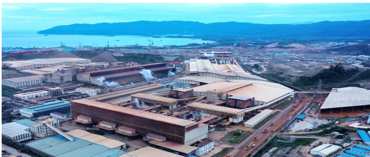
Hengjaya and Ranger RKEF operations
