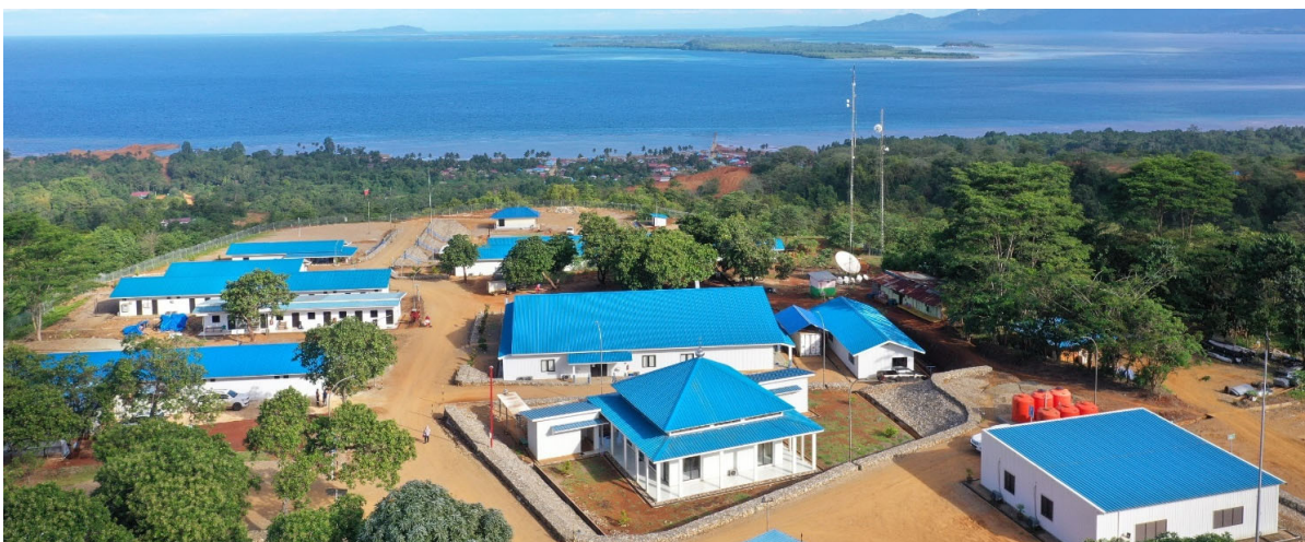
Site infrastructure including a mosque, sports facility and accommodation is now completed
