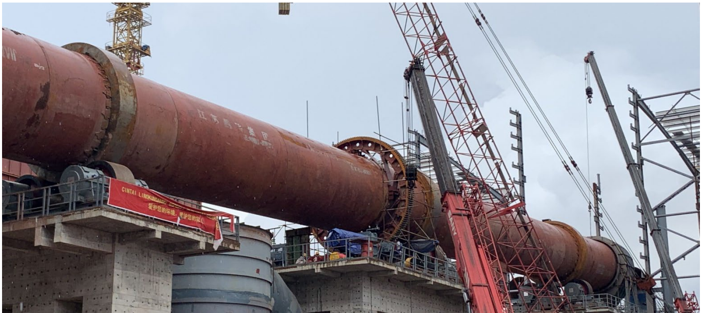
Oracle Nickel RKEF construction has advanced rapidly during the June quarter
