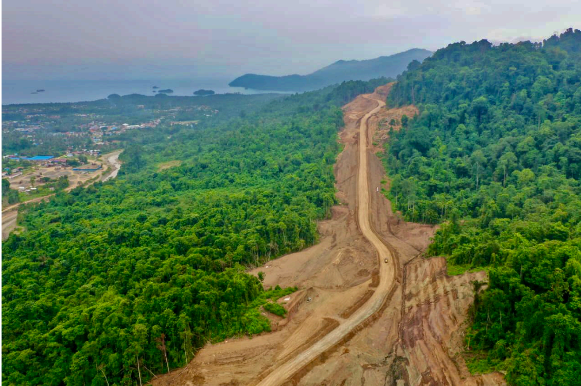
Haul road segment to IMIP river to IMIP is 95% complete
