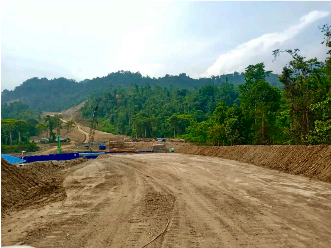
Abutments joining haul road to bridge and bridge construction
